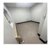
After: Removed tiles and installed drywall, new flooring, fresh paint, and ceiling grid/ lighting
